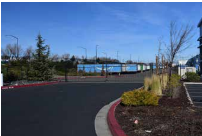
Gates visible from public areas are to be constructed of tubular steel or similar material
