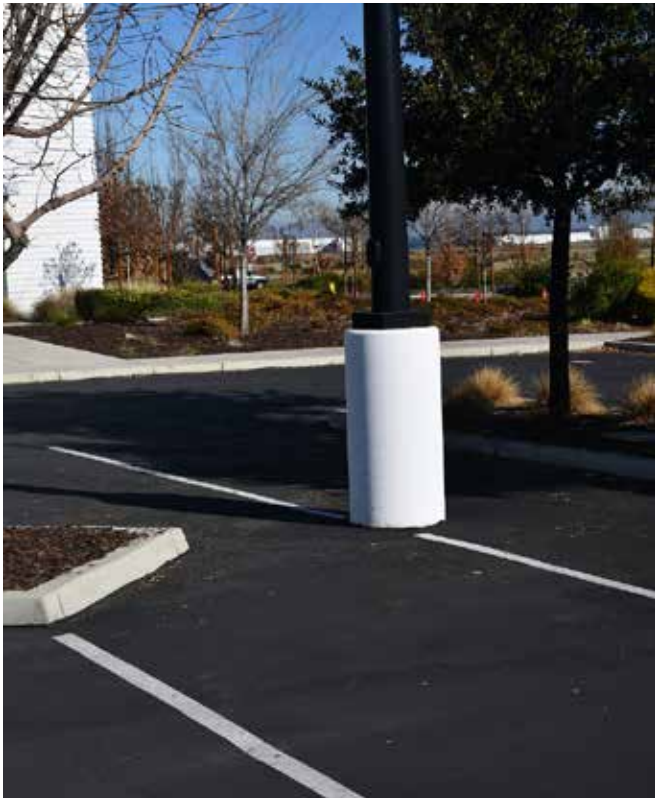
Light fixture bases should be protected
