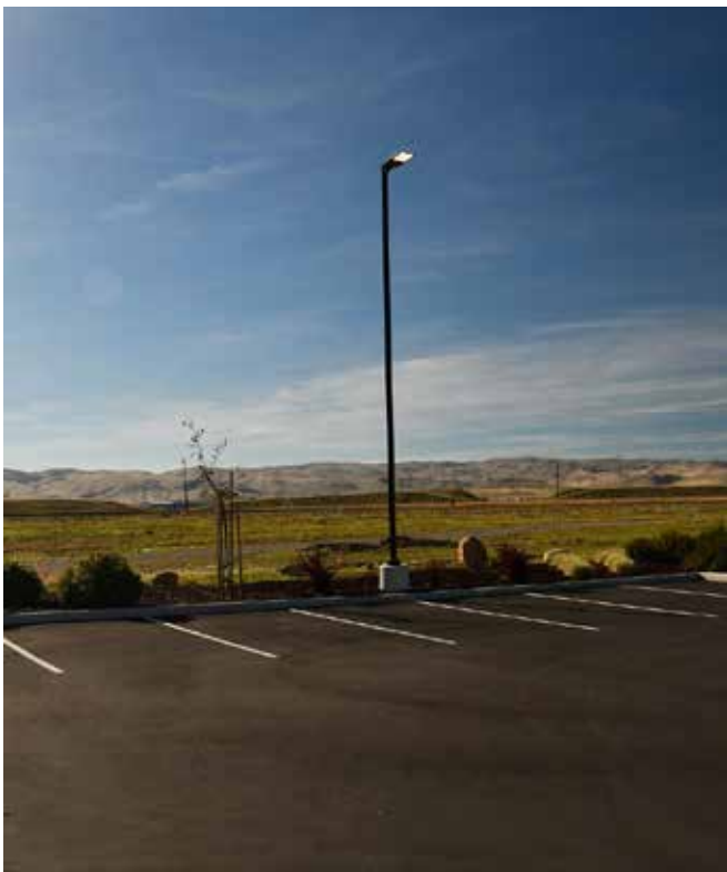
Typical parking lot lighting
