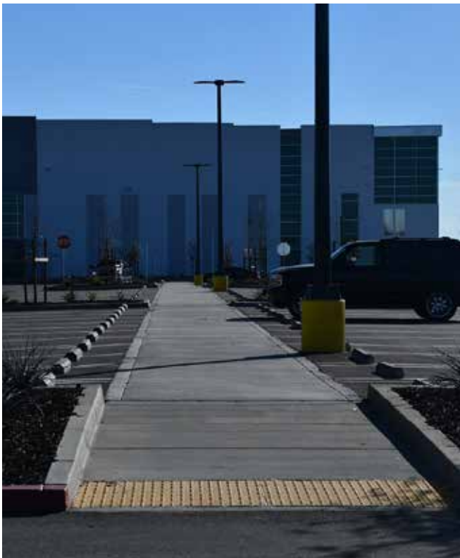
Pedestrian connections between building
