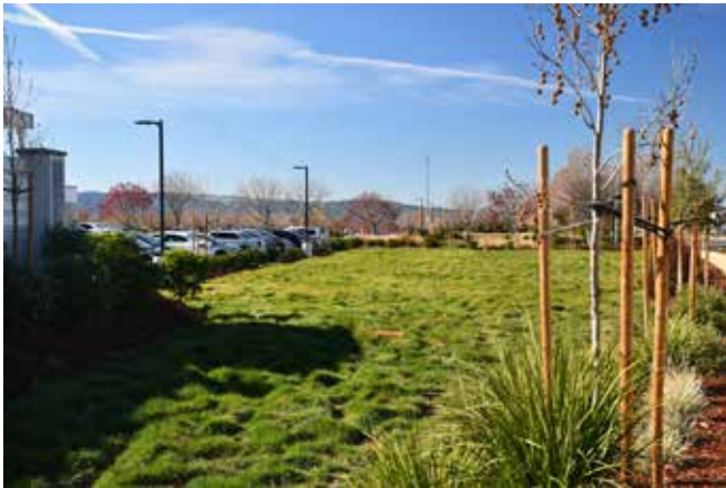
Typical bioretention planter
