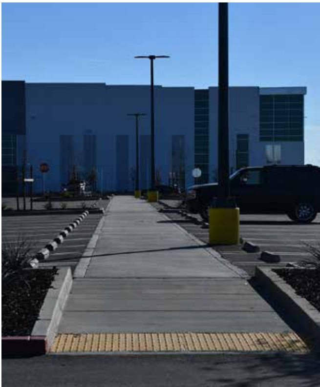
Pedestrian connections between building
