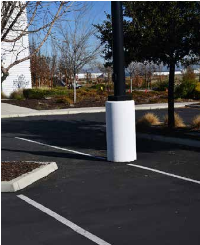
Light fixture bases should be protected
